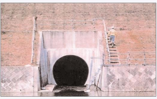
• Xypex Concentrate was applied to existing deteriorated concrete box culvert. Admix the was used in new tunnel lining.
