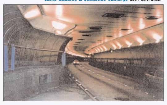
• The shotcrete lining of two parallel tunnels were treated with 2,600 sq. metres of Concentrate & Modified. Patch'n Plug was used to repair more than 1,700 defects in the concrete.
