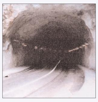
• Repair 30 year old, 105 m tunnel using Concentrate & Modified White. Old concrete was removed and replaced with shotcrete.
