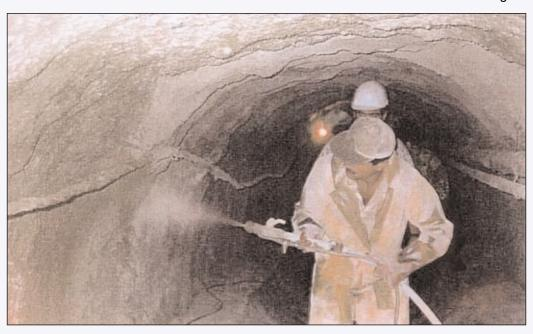
$\bullet$  Over 20,00 lbs. of Xypex Concentrate and Modified were spray applied to shotcrete. Stopped all water infiltration & provide protection to the concrete from H2S.
