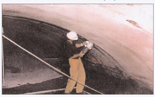
• Extensive crack repair using Concentrate & Patch'n Plug to seal water seepage.
